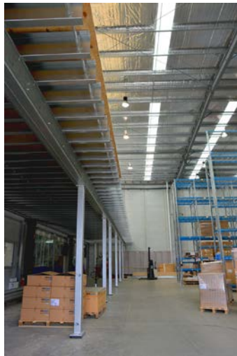
Figure 1: Construction Commences for ebm-papst A&NZ's Centre of Excellence
